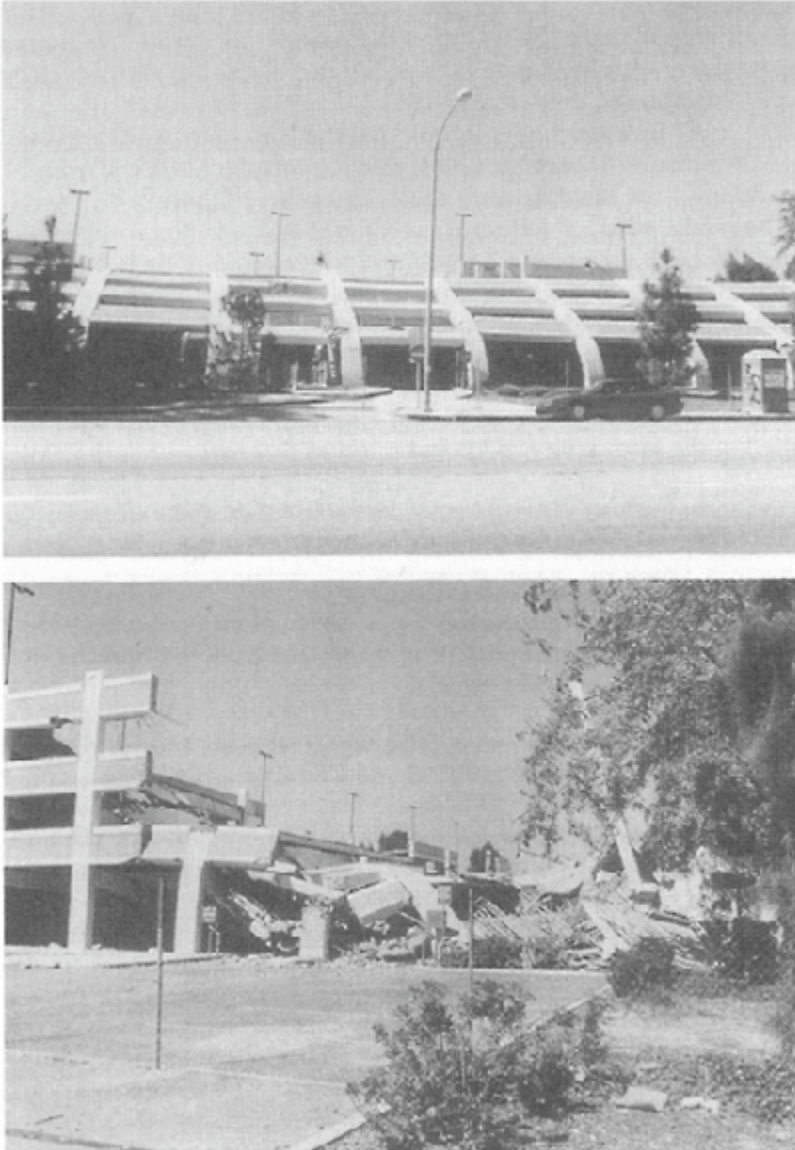
Figure 6.9. A CSUN campus parking lot shown before and after the 1994 Los Angeles earthquake. Fortunately, the earthquake occurred during a semester break, on a holiday, and very early in the morning. Photos by K.Fearn. Reprinted by permission.
